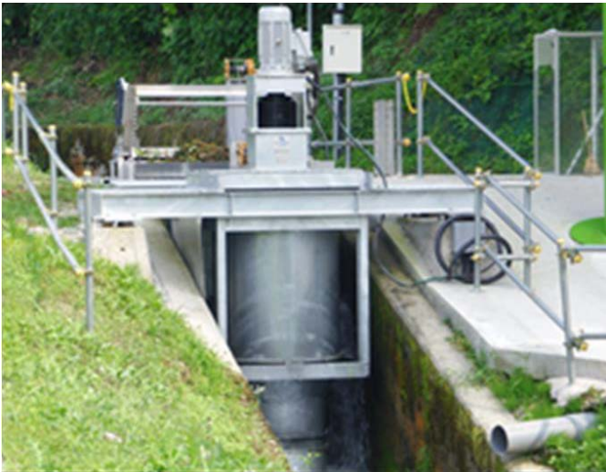
Micro Hydro 5kW ~ 50kW installed in Japan
