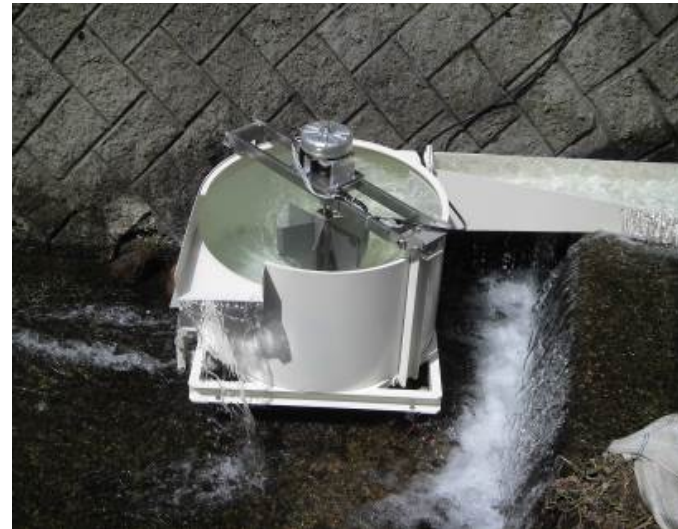
Micro Hydro 1kW ~ 15kW installed in Japan
