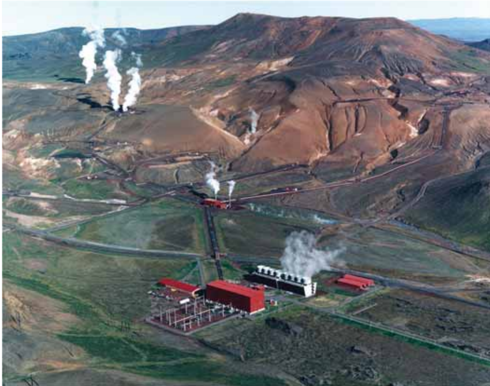
Figure 19: Krafla 60 MW Geothermal Power Plant in Landsvirkjun, Iceland
