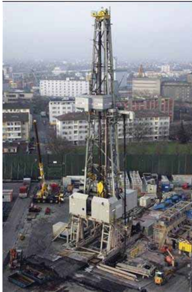
Figure 17: Heavy Drilling Rig in Switzerland
