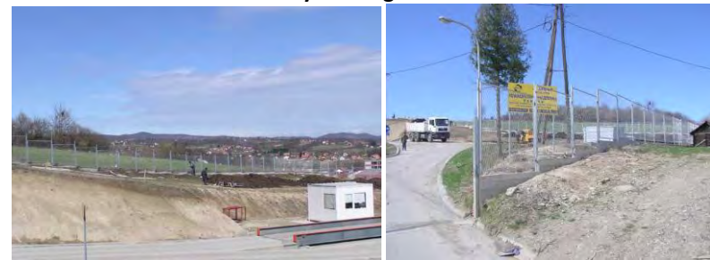
Security Fencing in Ramichi
