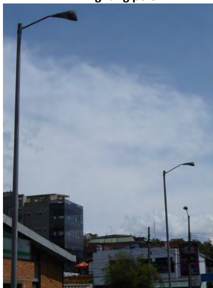
LED lighting pole
