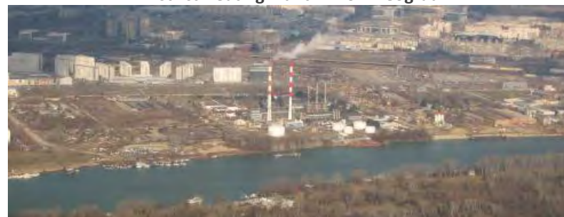
District Heating Plant in Novi Beograd
