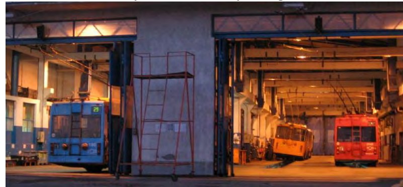
Trolleybus Maintain Shop in Belgrade
