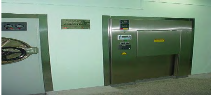
Figure 29: Newly replaced hospital equipment
