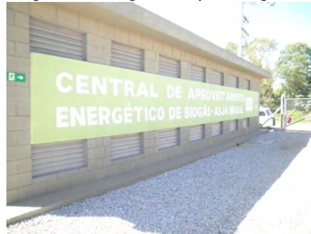
Figure 17: SLU's Biogas Electricity Generating Plant
