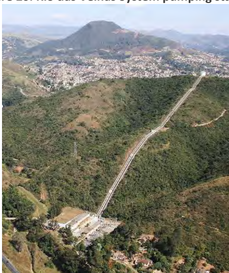
Figure 20: Rio das Velhas System pumping station
