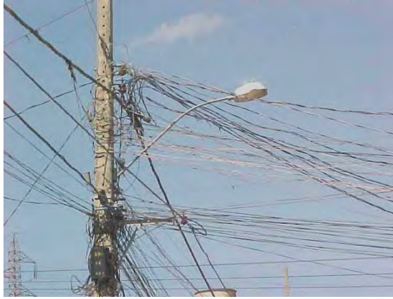
Figure 27: Illegal electricity connection in favelas
