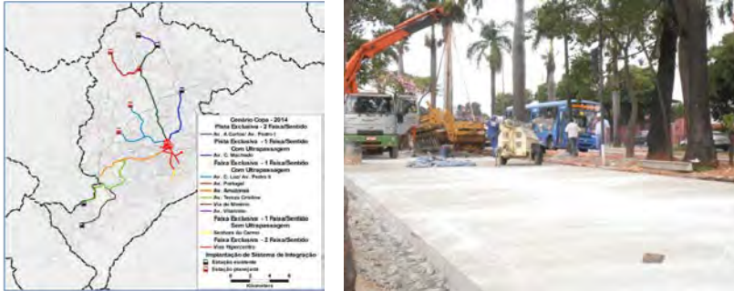
(left image) Belo Horizonte's BRT construction plans (right image) One of many BRT construction sites in Belo Horizonte
