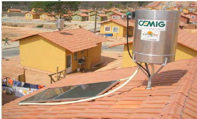
Figure 30: Solar water heater
