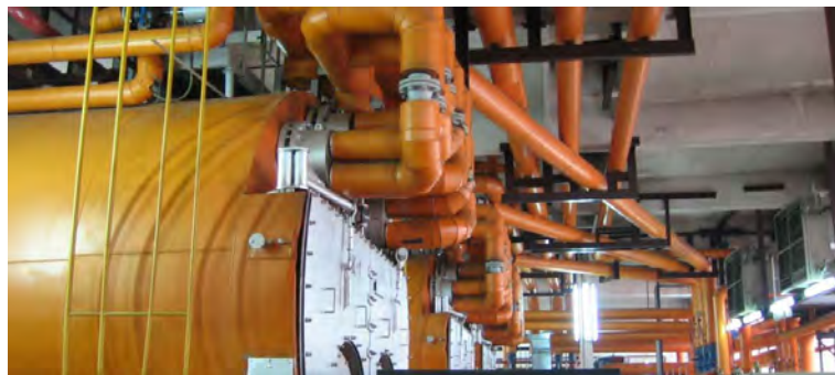
Hrasno Boiler House
