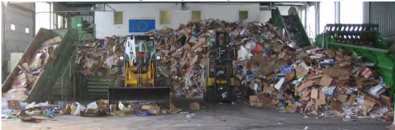
Sorting Facility at Sarajevo Landfill
