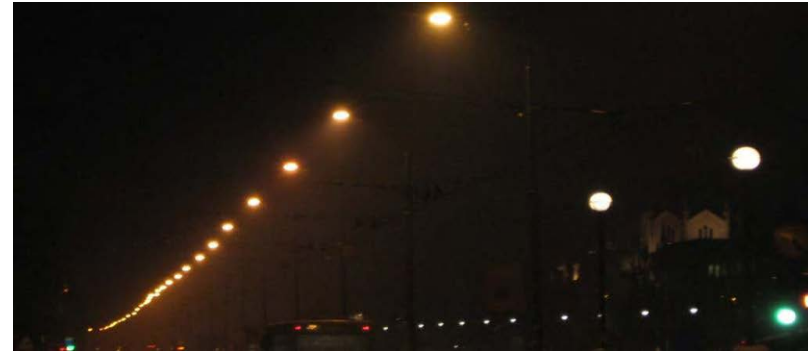
Street Lighting on Hiseta Ulica
