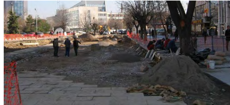
Extension of Pedestrian Path
