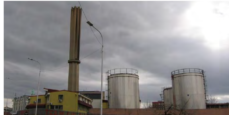
Termokos Plant and its Mazut Containers
