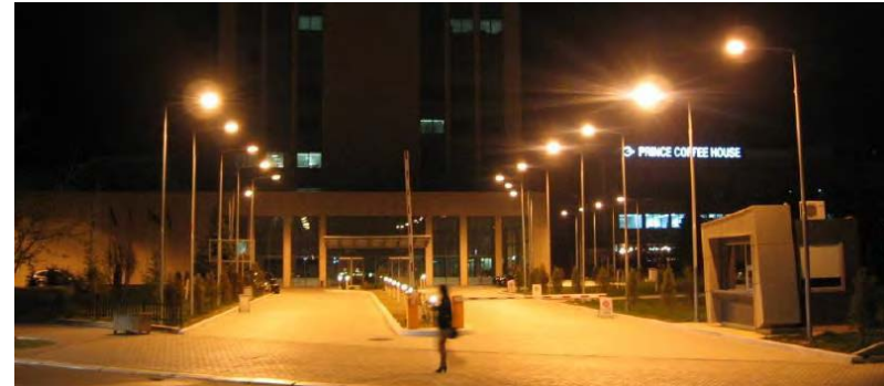
High Pressure Sodium Street Lights in Pristina
