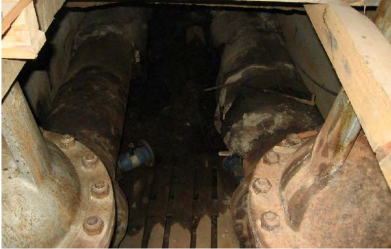
District Heating Piping with Classic Insulation, in Pristina
