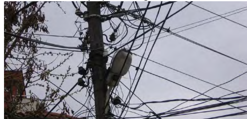
Mercury Vapor Street Light in Pristina
