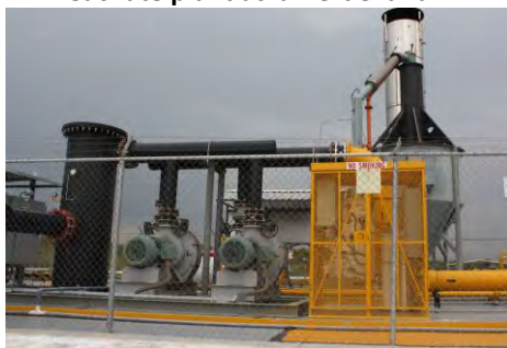
Leachate plant at la Verde landfill
