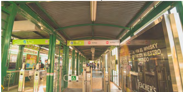
BRT bus stop in León
