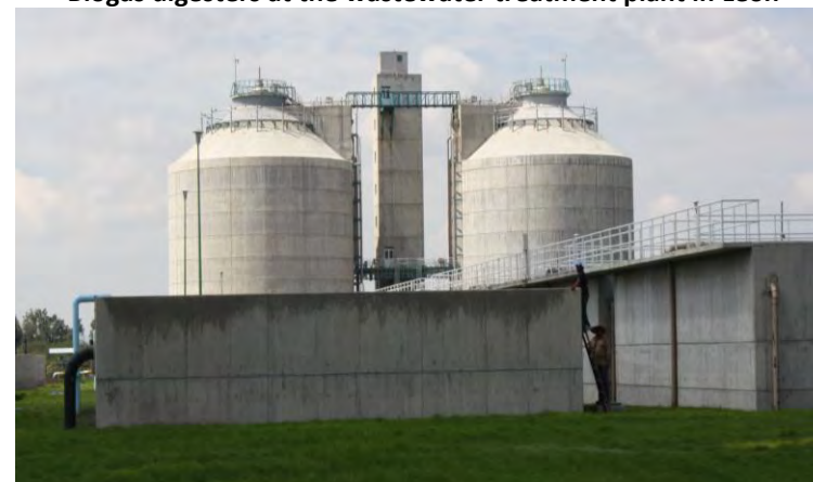
Biogas digesters at the wastewater treatment plant in León
