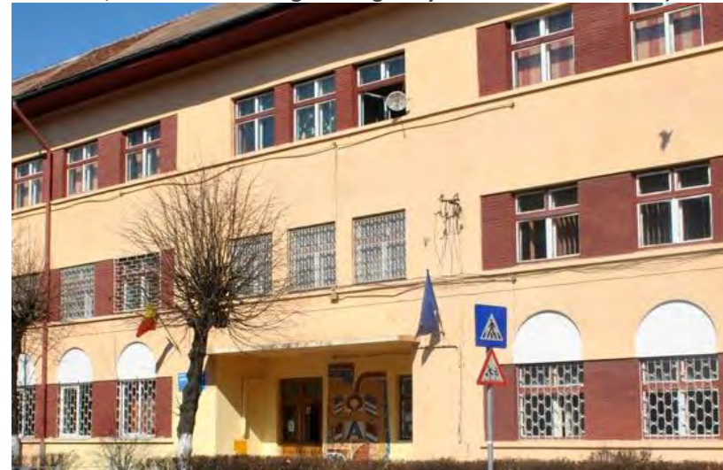
School 13, one of the buildings managed by local authorities in Brașov
