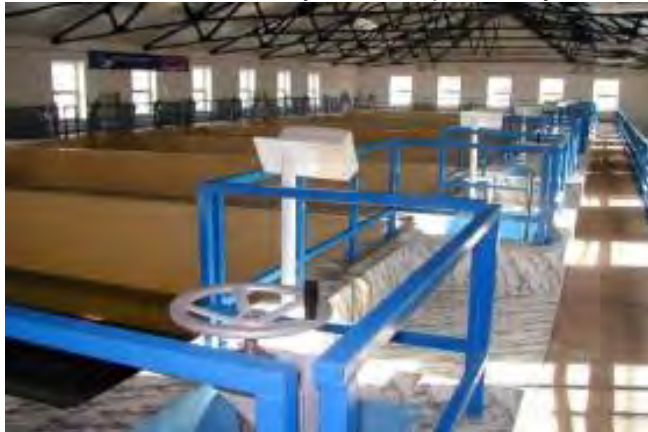
Water treatment plant in Braşov County
