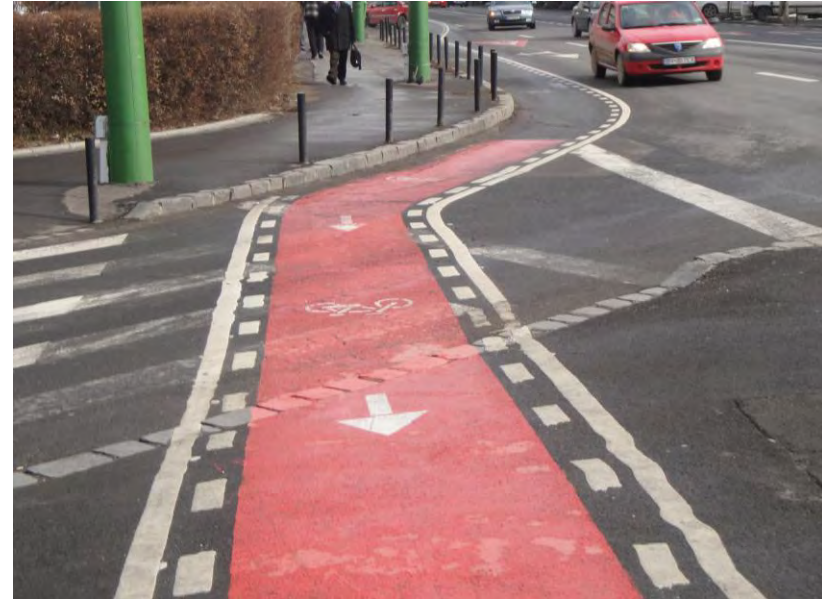
Bike lane in Braşov
