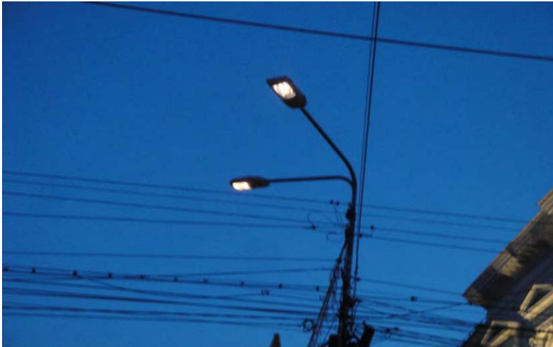
Lighting pole with vapor sodium lamps
