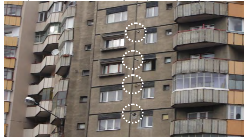
Chimneys from individual micro-heating units, protruding through outer walls
