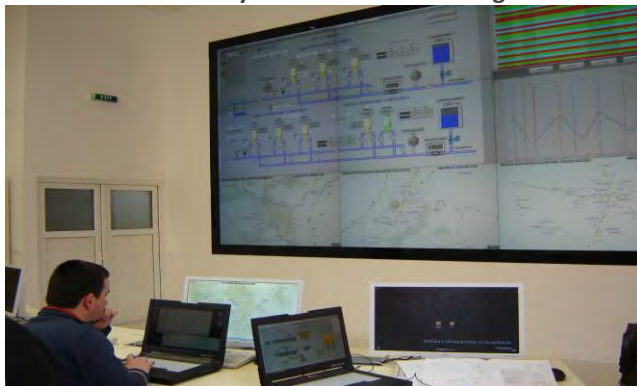
SCADA system water monitoring
