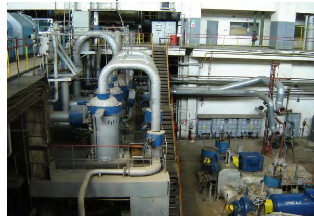
CET Iași has been modernized
