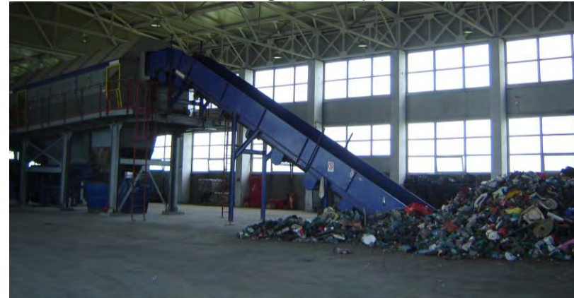
The sorting station at Țuțora landfill
