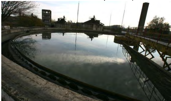
Wastewater treatment plant in Iași
