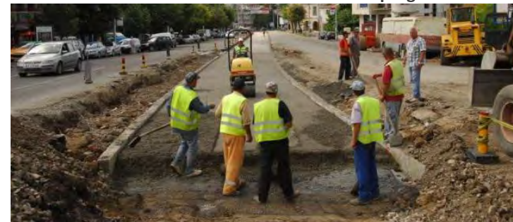
Tram network modernization work in progress
