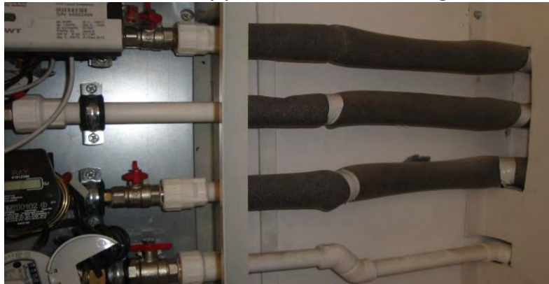
Horizontal distribution pipe in a rehabilitated building in Craiova
