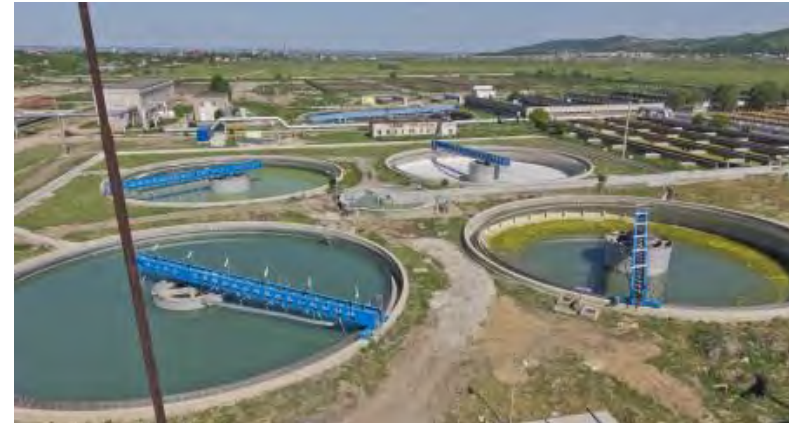
The water plant in Iași has been modernized with ISPA funds
