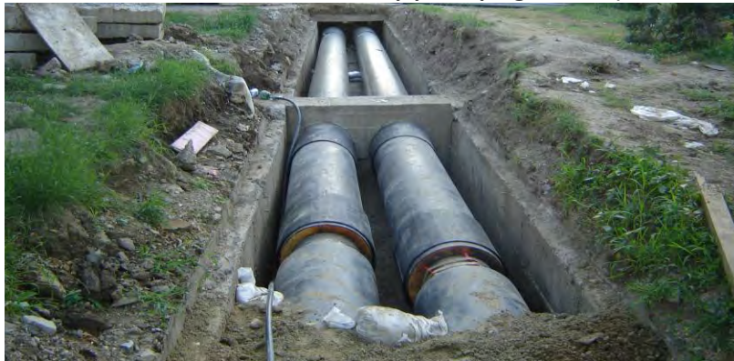
Rehabilitation of hot water pipes in progress in Iași
