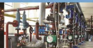
Power and Heat
