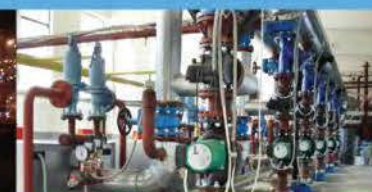
Power and Heat
