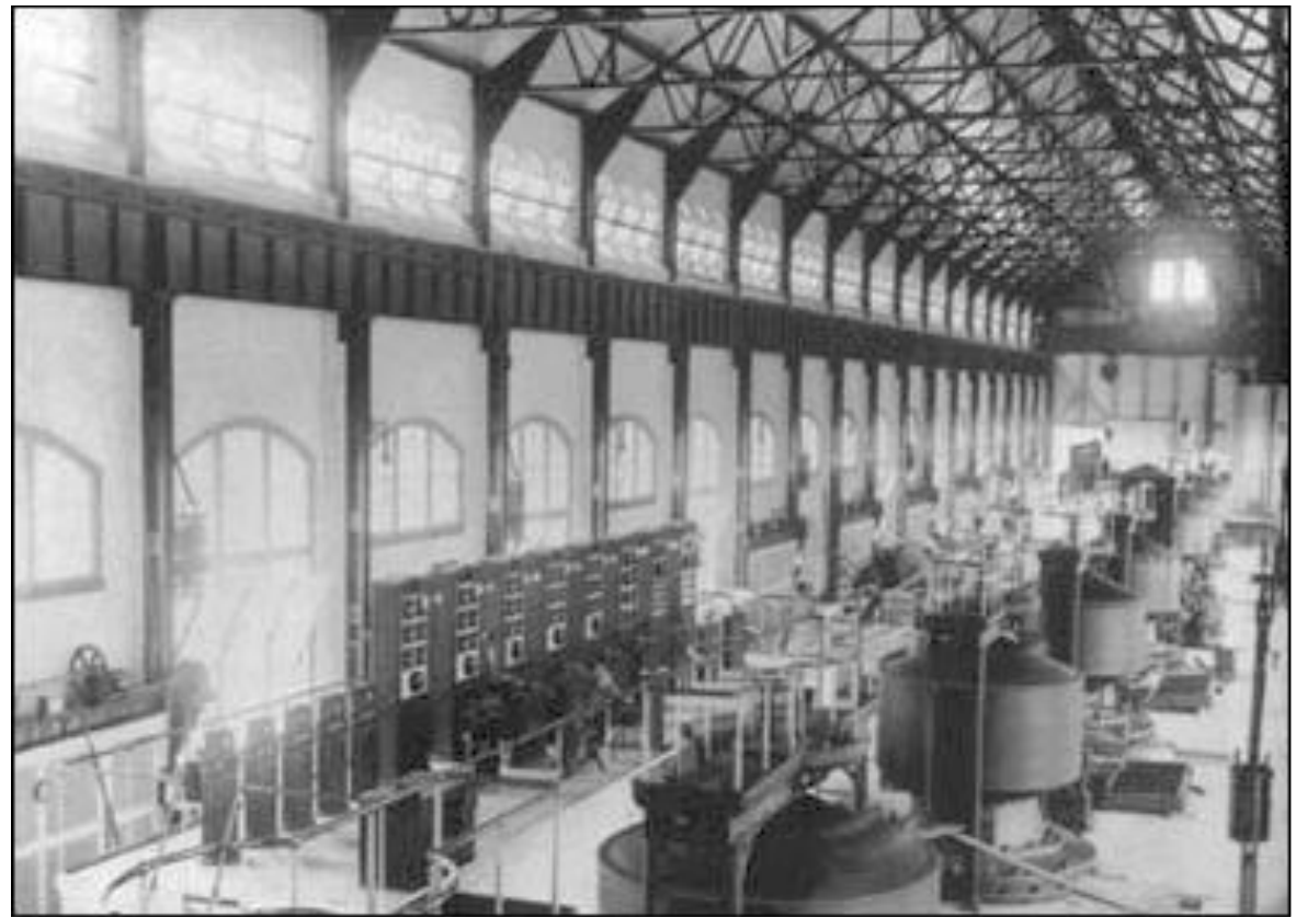
Niagara Power Station
