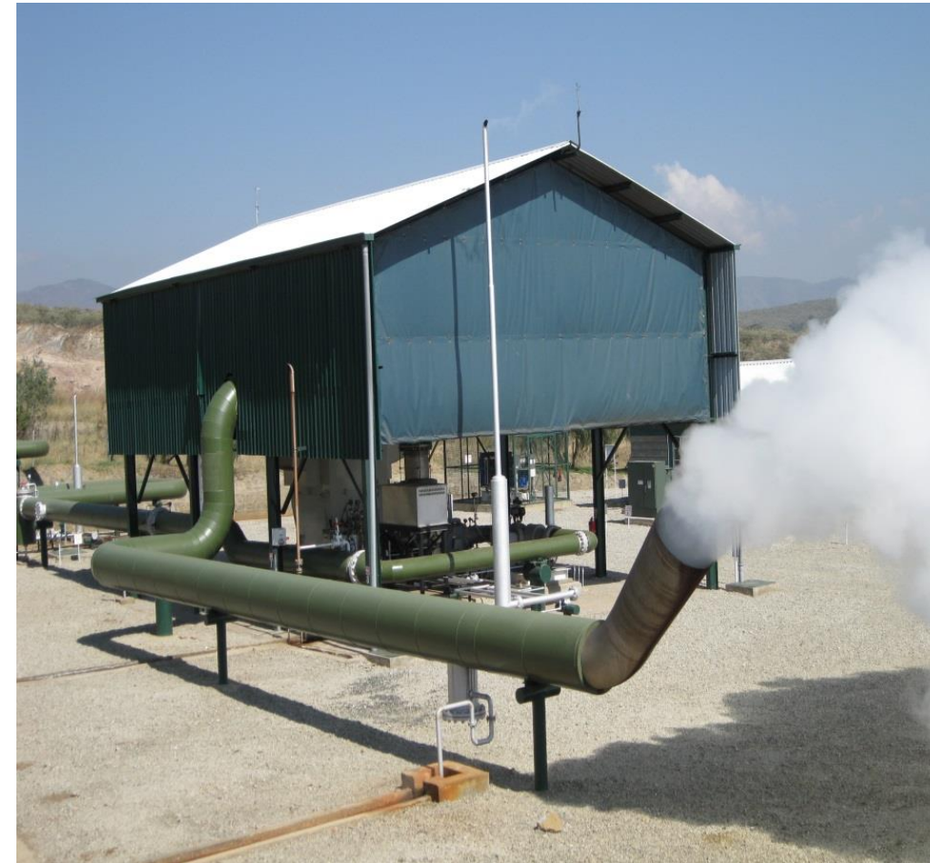
1.4Mw Back Pressure Plant.
