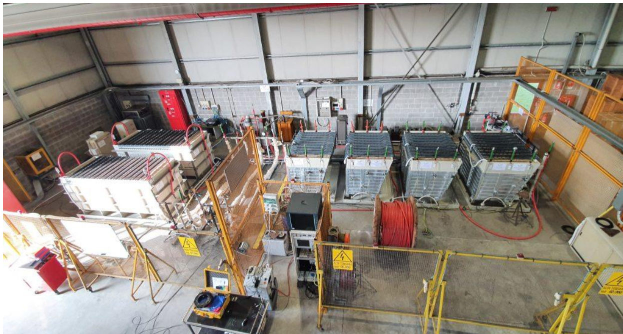
Image of RSE's MV Cable Diagnostics Laboratory.
