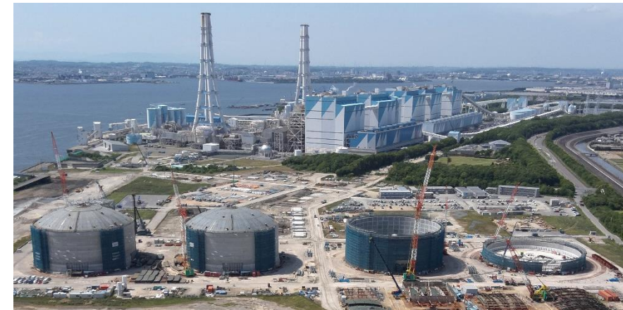
Construction site view (as of Mar. 2026)
