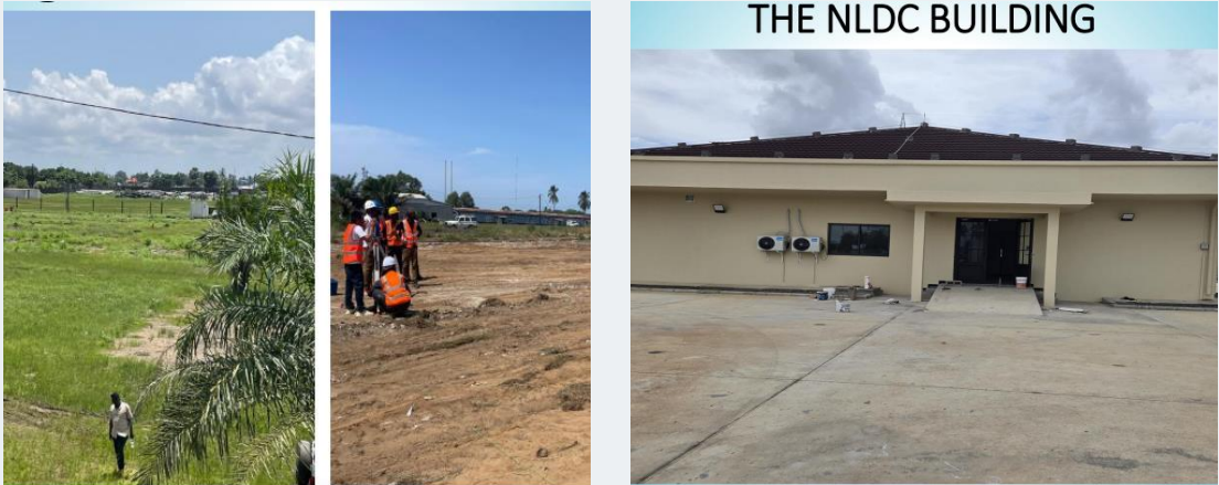
Top: LEC staff at the National Control Center. Below: NLDC site in March 2025 and the completed NLDC building.
