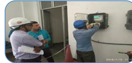
HOTT - Practical exposure of working on live DT meter
