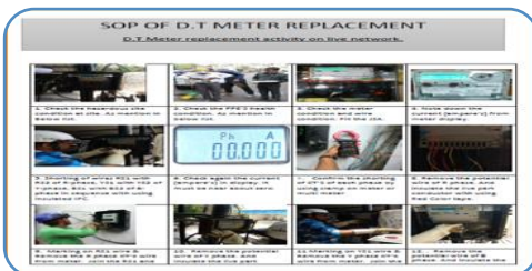
SOP for online DT Meter Replacement
