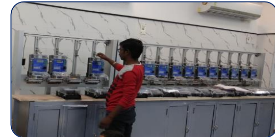
In-house Test Bench- 02 Nos-15 position Single Phase & One 15 position Poly phase
