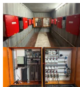
Figure 7 – Control & Communication Systems and Lithium Ion battery banks
