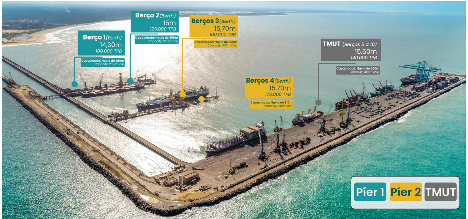
Figure 3. PECÉM port and port infrastructure
