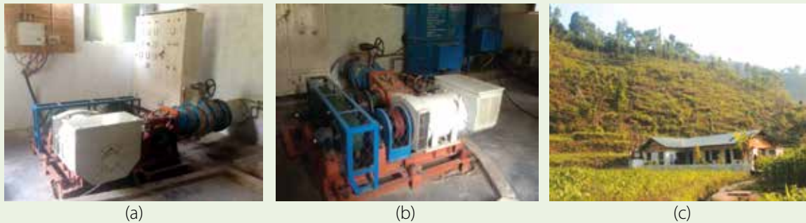
Figure A2.11 (a) Powerhouse (b) Turbine and generator set (c) Control panel and the MHP system of Giringdi Kholan MHP
