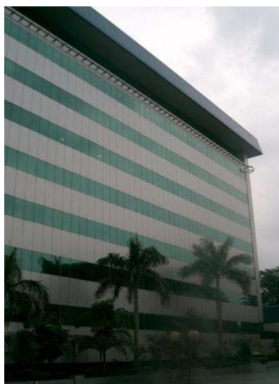
Figure B-1: PLN Building No. 1
