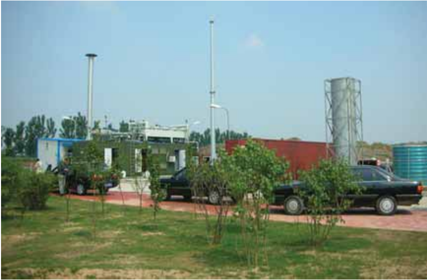
Figure 13.5 Landfill Gas Processing Facility at the Tianjin Shuangkou Landfill
