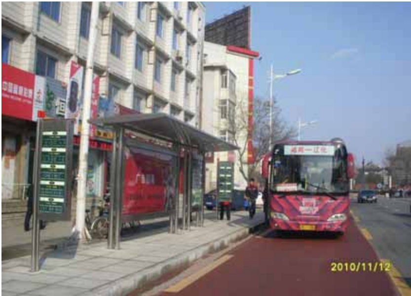
Figure 11.3 Bus Priority Lane in Liaoyang, Liaoning Province
