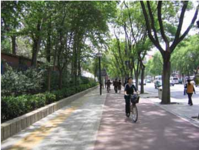
Figure 10.2 Integrating Cyclists with Pedestrians Using Different Colored Pavement in Xian
