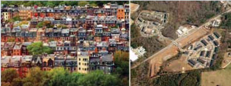
Figure B4.6.1 Traditional Grid of Back Bay, Boston (left), Compared with a Cul-de-sac Layout
