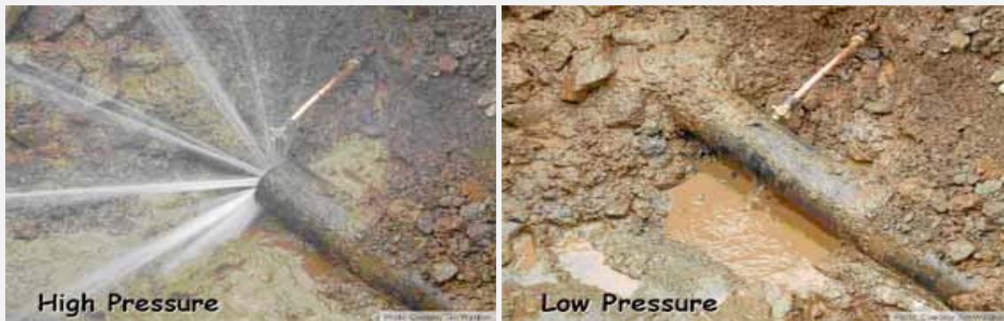
Figure 1: The difference in water losses when water pressure is reduced.
