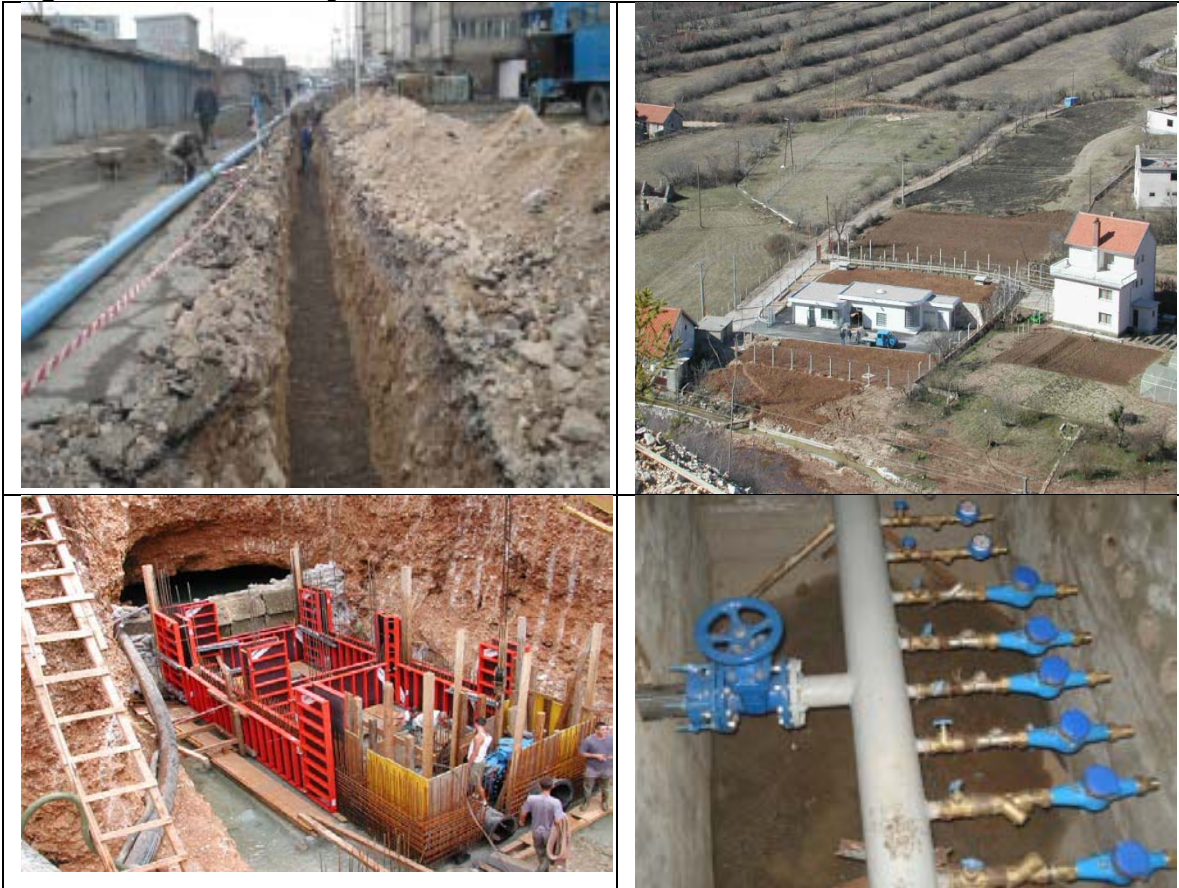
Figure 1. Photos of Project Execution
