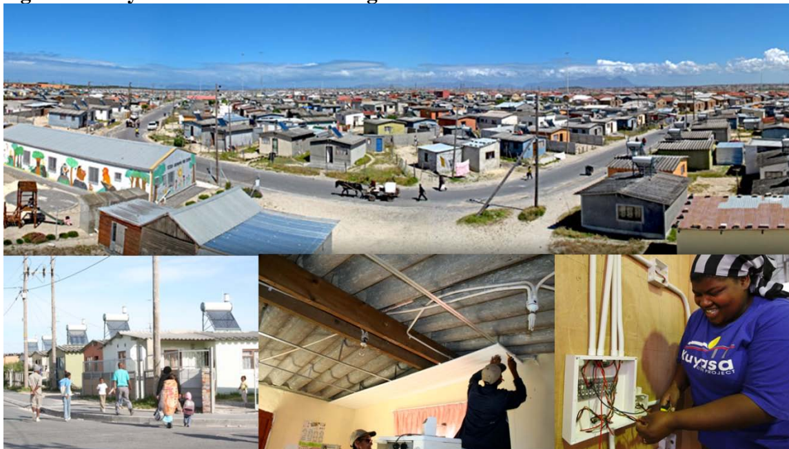
Figure 2: Kuyasa Low-Income Housing - Installation of EE Measures
