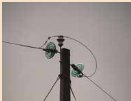
Box figure 2.1.1 SWER line, New Zealand
