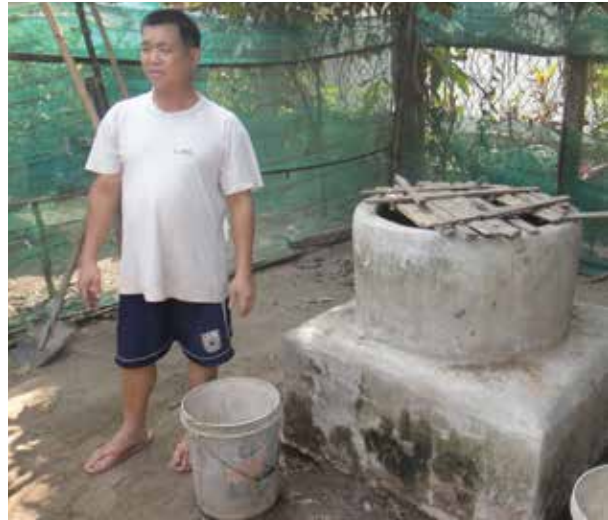
Inlet for feeding slurry into the household biodigester, Sikhottabong District, Vientiane capital
