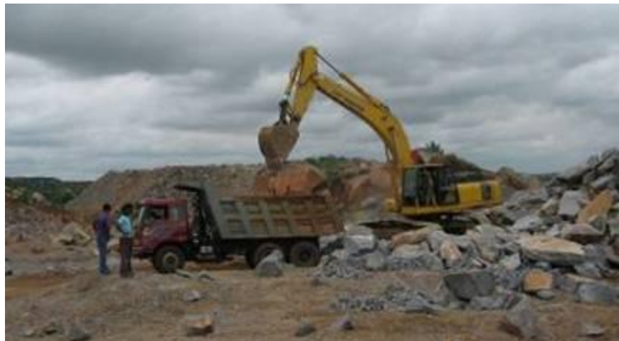
Hydraulic excavator feeding a truck to transport excavated materials
