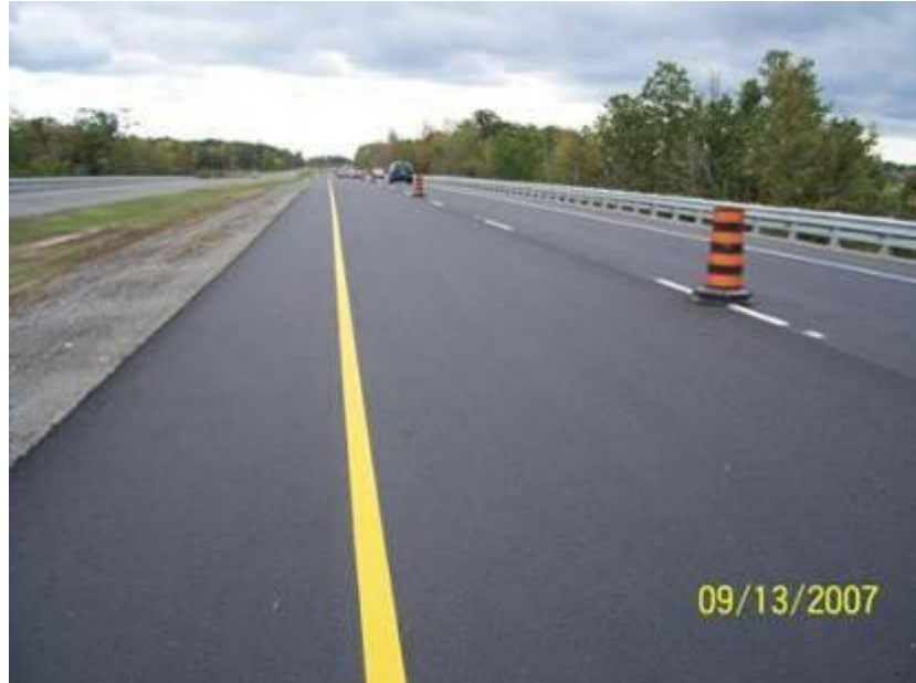
Perpetual pavement on the Highway 406, Ontario, Canada ( www.mto.gov.on.ca )
