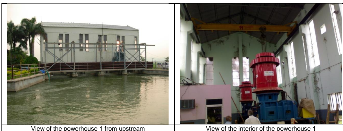
Photo 6-1 View of Adanki Branch Canal Powerhouse 1
