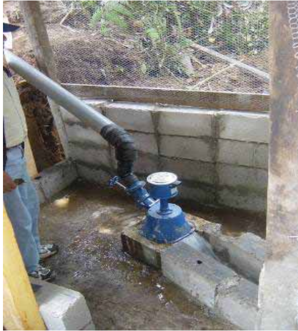
Photo 2.2: Vietnamese 200 watt, medium-head picohydro “turgo” unit in Ecuador
