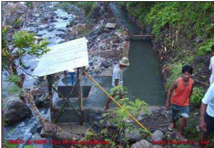
Photo A2.4: Igputoy Picohydro System for Community Electricity Supply, Antique Province (Solar Electric Co. Ltd.)
