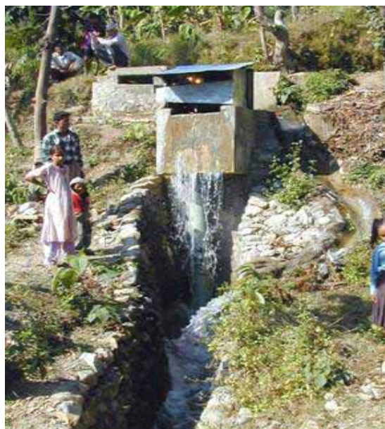
Photo A1.4: PT1 Installation in Operation
