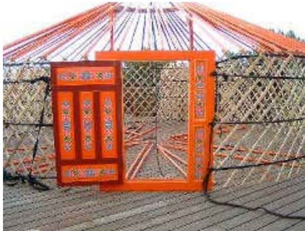
Figure 2.2: The Wooden Support Structure of a Ger, Showing the Door and Frame, Walls, Rafters, Roof Ring, and Belly Bands
