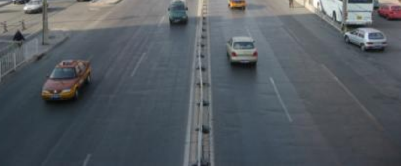
Two way 6-lane road (The special lane is on the right side)
