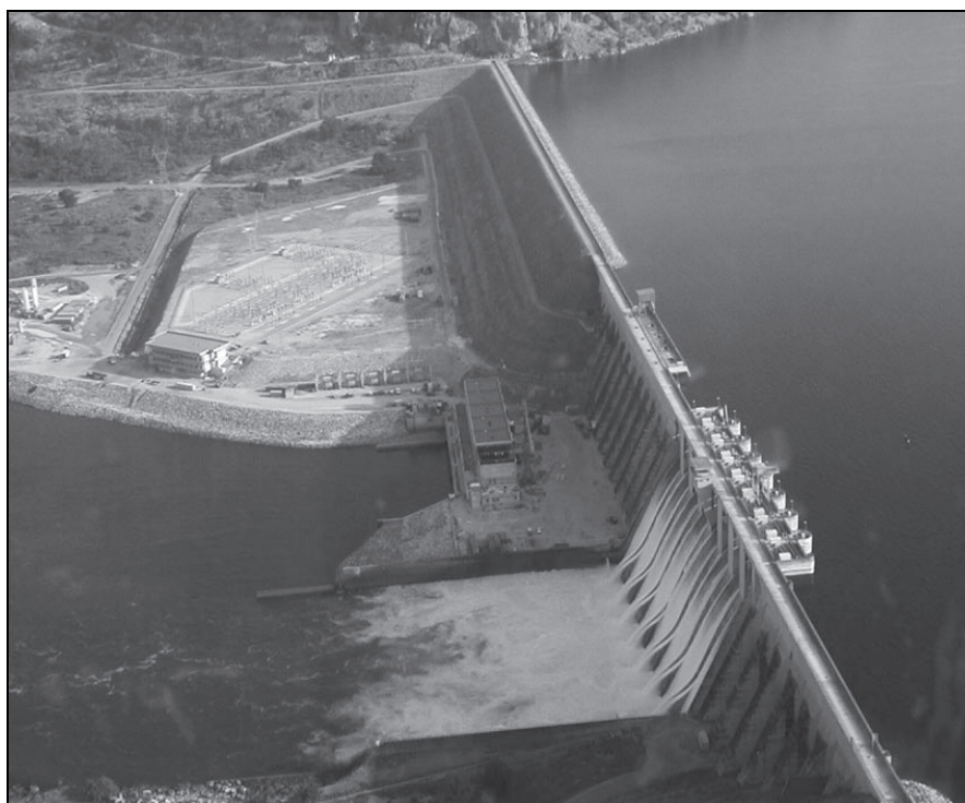
Figure 3 Aerial View of the Manantali Dam
