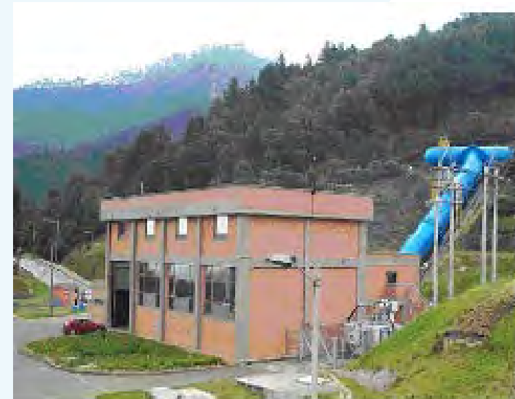
Santana micro-hydroelectric plant
