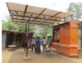
Solar PV power station for the Entasopia micro-grid, Kenya
