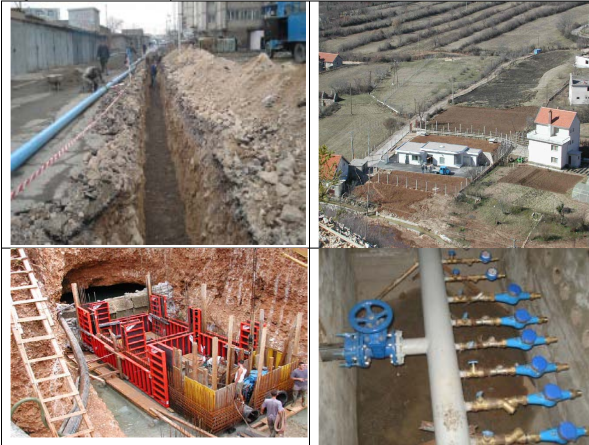
Figure 1. Photos of Project Execution
