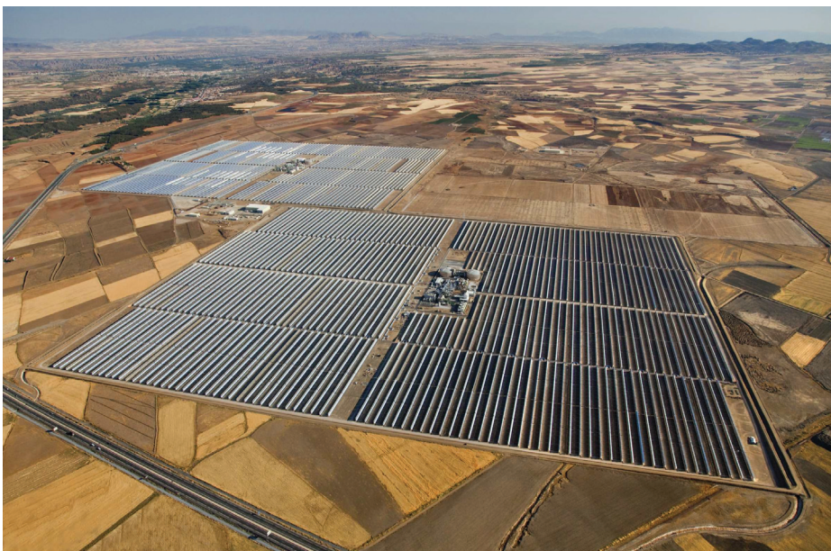
Figure 1.3 ■ Parabolic Trough Power Plants Andasol 1 (front) and Andasol 2 (rear) in Spain with a Capacity of 50 MW Each and a Storage Size of 7.5 Full-Load Hours. The Power Block and the Storage are in the Center of Each Solar Field
