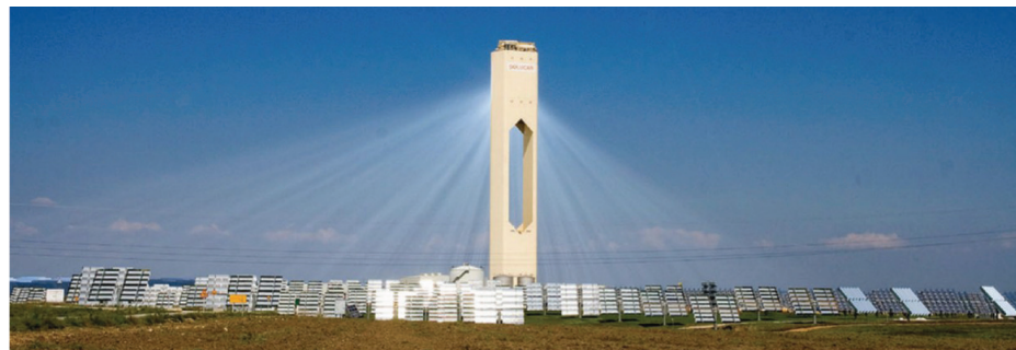
Figure 1.7 ■ 11 MW el Power Tower by Abengoa, Hundreds of Heliostats Concentrate the Sun (up to 500 Times) Onto an Absorber on the Top of the Tower
