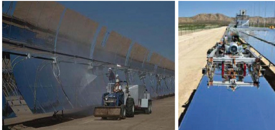
Figure 1.31 ■ Left: Conventional Cleaning Methods (Cohen, 1999), Right: Water-Efficient Cleaning Using a Cleaning Robot of Fresnel Collector by Novatec Biosol (Novatec, 2010)
