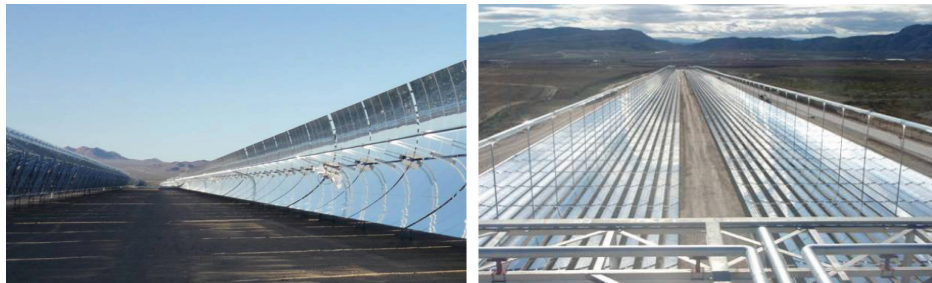
Figure 1.1 ■ Line-Focusing Systems: Left: Parabolic Trough Collector: 64 MW el Power Plant Nevada Solar One; Dimensions: Collector Aperture Width 5 m (Morin, 2010). Right: Linear Fresnel Collector: 1.4 MW el Plant PE1 in Murcia, Spain; Dimensions: Receiver Height Above Mirror Field: 7 m (Novatec, 2010)
