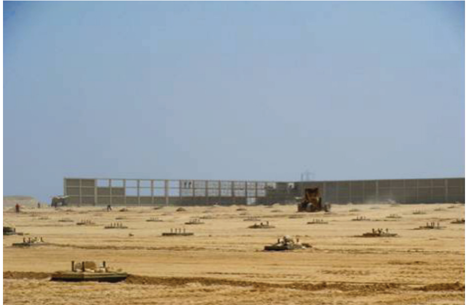
Figure 1.15 ■ Construction Site of Parabolic Trough Solar Field At Kuraymat (Egypt) with the Foundations of the Solar Field
