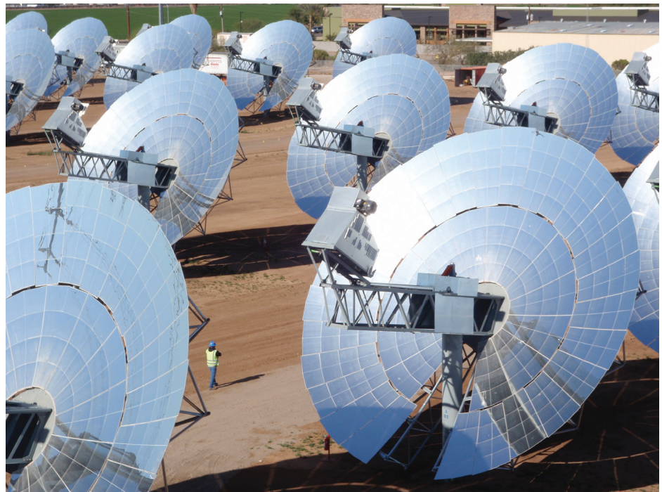
Figure 1.8 ■ Maricopa Dish Stirling Farm in Arizona, the Park has a Rated Power of 1.5 MW el Consisting of 60 Dish-Stirling Units
