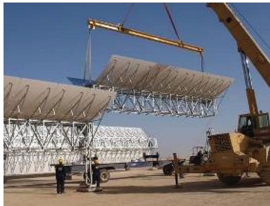
Figure 2.8 ■ Installation of Mirror Collector at Kuraymat Site
