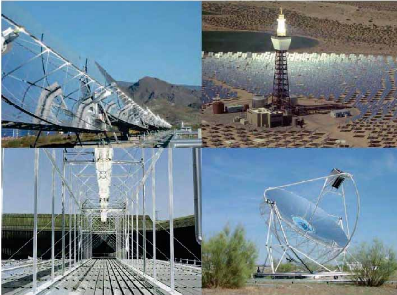
(a) Parabolic trough system (b) Linear Fresnel reflector (LFR)
