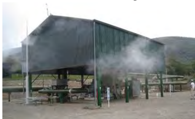
Figure 4-5 Weather shield over a turbine at the Olkaria field in Kenya
