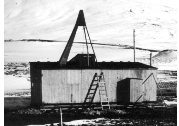
Drilling in Laugarnes
