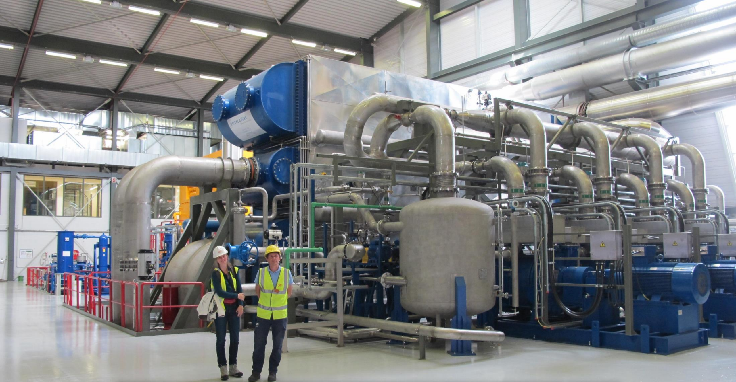
Gas and condensation water are taken from one of the turbines at Hellisheiði
