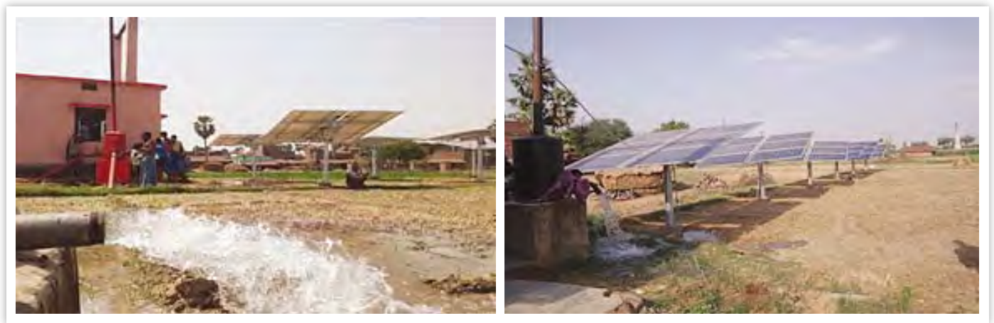
Control module monitoring.
