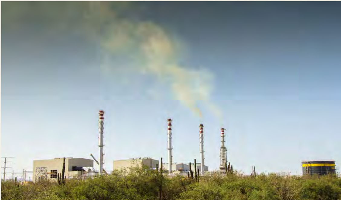
Bunker oil Power Facility Baja California Sur
