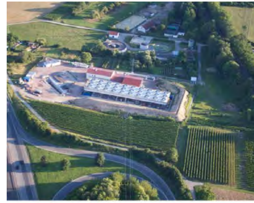
EGS at Insheim, Germany, 4.3 MW, air-cooled DEC
