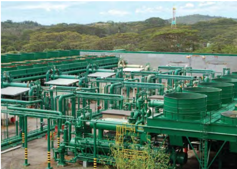
Puna, Hawaii, USA, 38 MW, 1992, 2004, 2012 (GCCU and air-cooled OEC)
