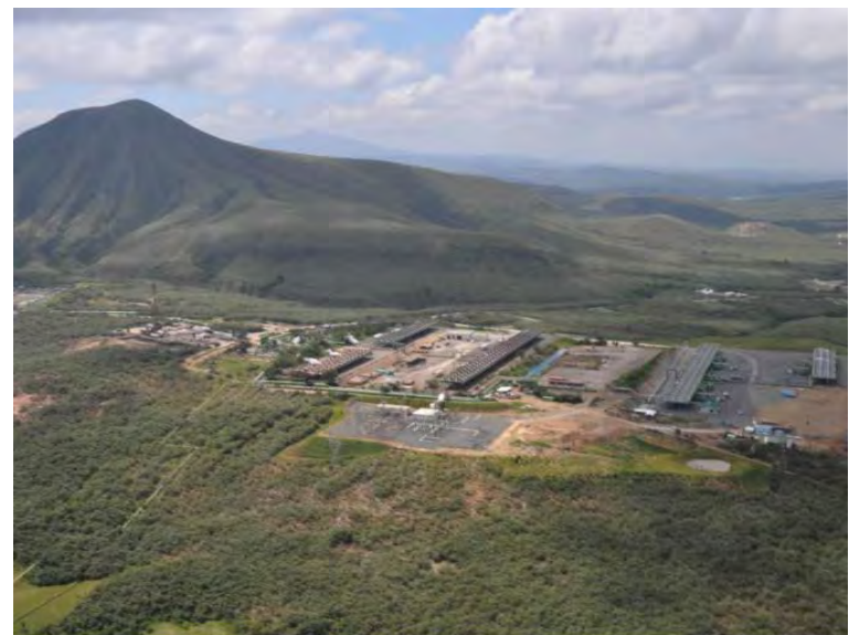
Olkaria III Complex, Kenya, 110 MW, 2000, 2008, 2013 (air-cooled OEC)
