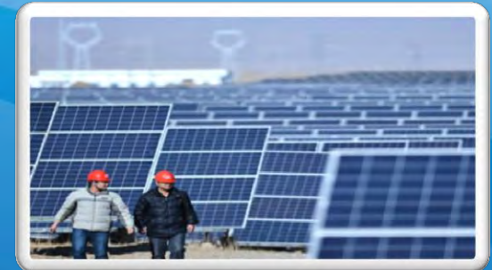
Solar power base in longyang Xia, Qinhai
