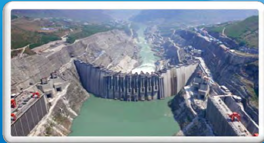
Xiluodu hydropower Station in Yunnan
