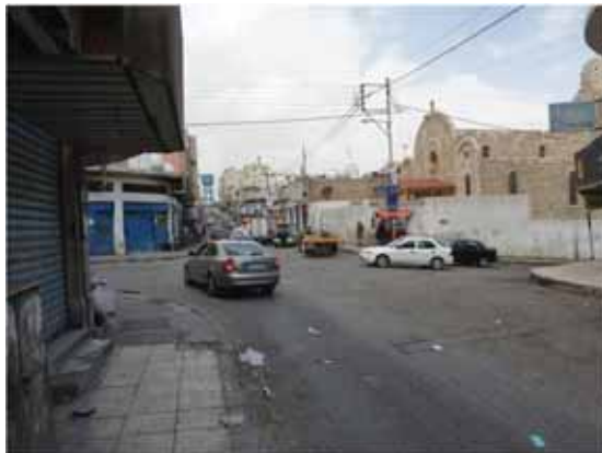
Poor Quality Footway
