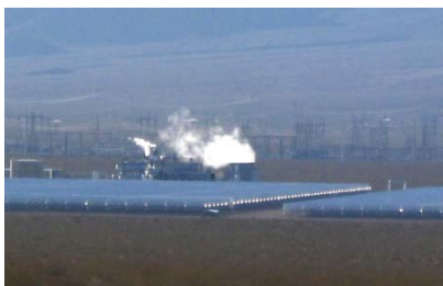
Figure a. Wet cooling at Nevada Solar One CSP plant ( http://www.basinandrangewatch.org/Water.html )
